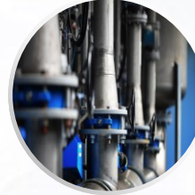
Valve Repair's - Workshop/On-Site (All Brands)
