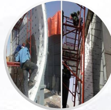
Insulation Services for GT & ST. Including other Major Equipment's
